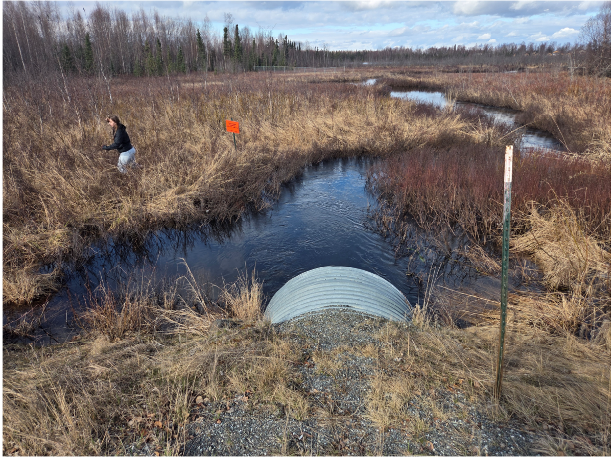
Figure 3-3. Horseshoe Lake Outlet Channel
