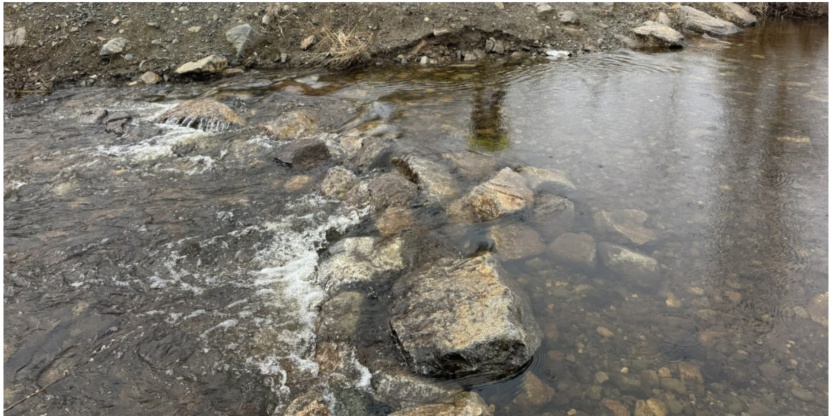
Figure 3-2. Rock Weir at Upper Caswell Lake
