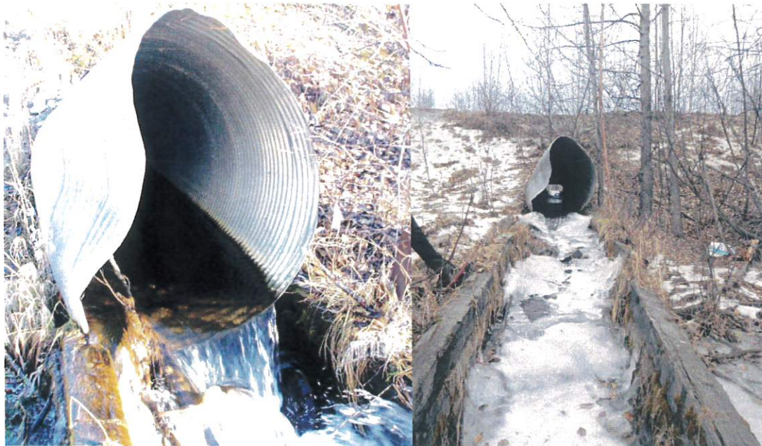
Figure 1. Site 20501156, located at the uppermost crossing of Crocker Creek on Settler's Bay Road, showing the perched and damaged culvert and collapsing fish ladder. This site is a total barrier to fish passage but salmon are recorded as using the upstream habitat prior to installation of the road and while the fish ladder was functional. Replacing this culvert and the fish ladder with a fish friendly structure and reconstructing the downstream channel will allow sockeye and coho salmon to return to habitat they are currently extirpated from.
