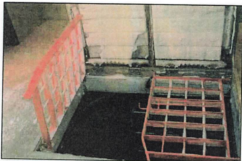
Before the upgrade, access to lift stations could be covered by deep snow in the winter. The borough had the main lift station moved out of the street and sheltered in a small, hoist-equipped building also housing the MultiTrove control panel.
