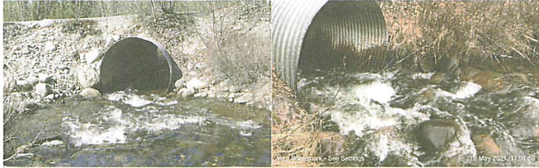
Figure 2. Site 20501470 showing the constriction of flow at the culvert and the high flows and sediment wedge at the inlet. This site is located at a tributary to Birch Creek near Talkeetna and impedes access to approximately 6.5 km of mapped stream habitat and extensive wetlands in an entirely undeveloped area.
