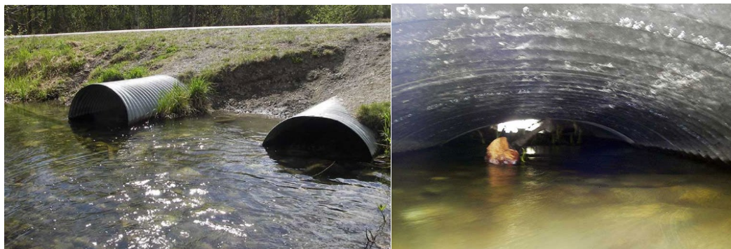
Figure 2. Photos of Site 20401288 near Neklason Lake showing the hydraulic flow exceeding capacity of the culverts
