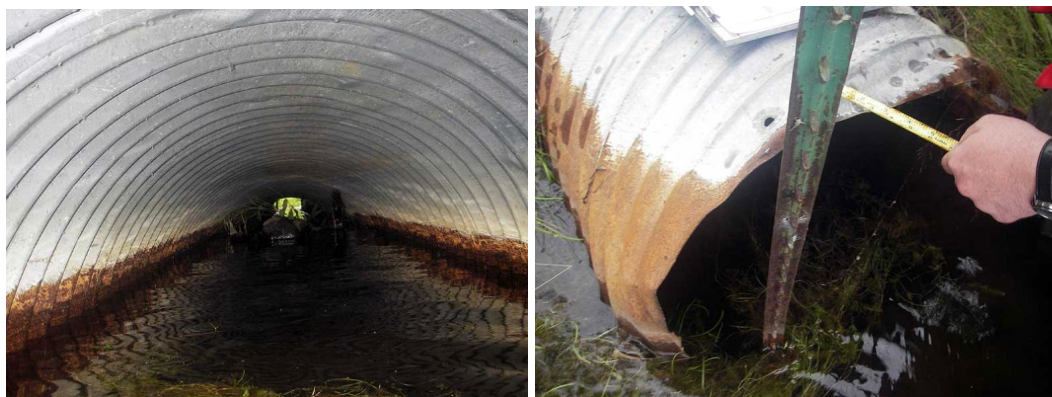
Figure 3. Photos of Site 20501436 showing the corroded culvert under Beaver Lake Road
