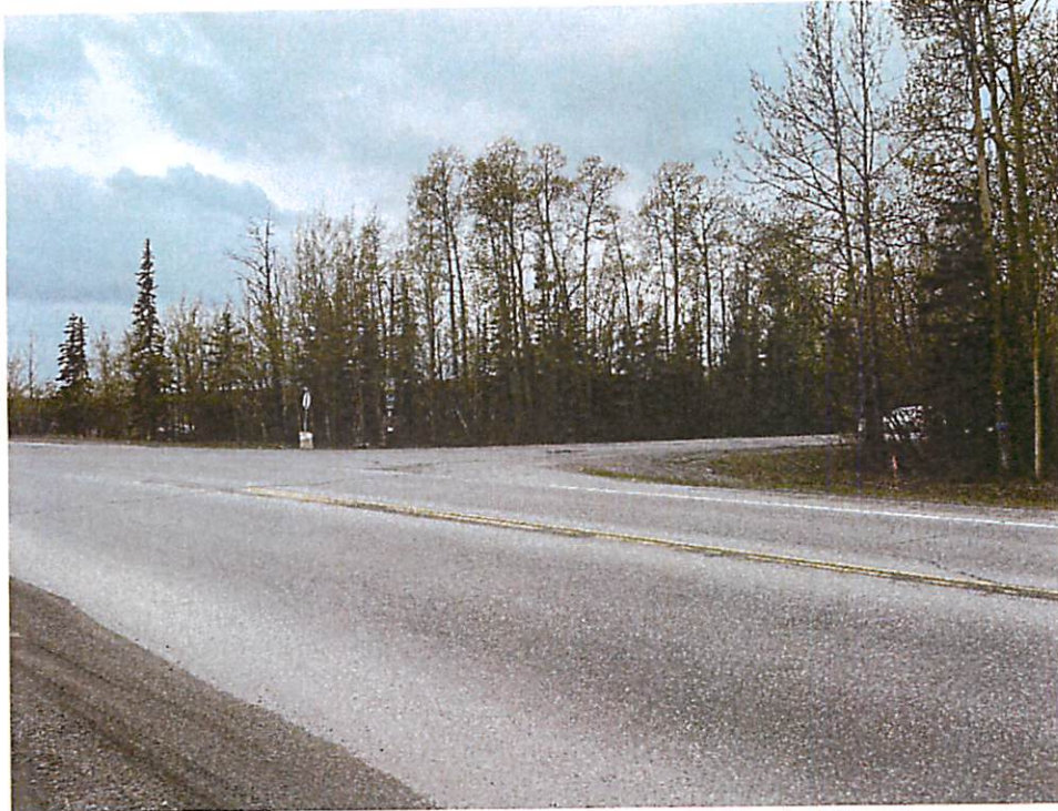
Photo 3 – Intersection of Tait Drive with Bogard Road
