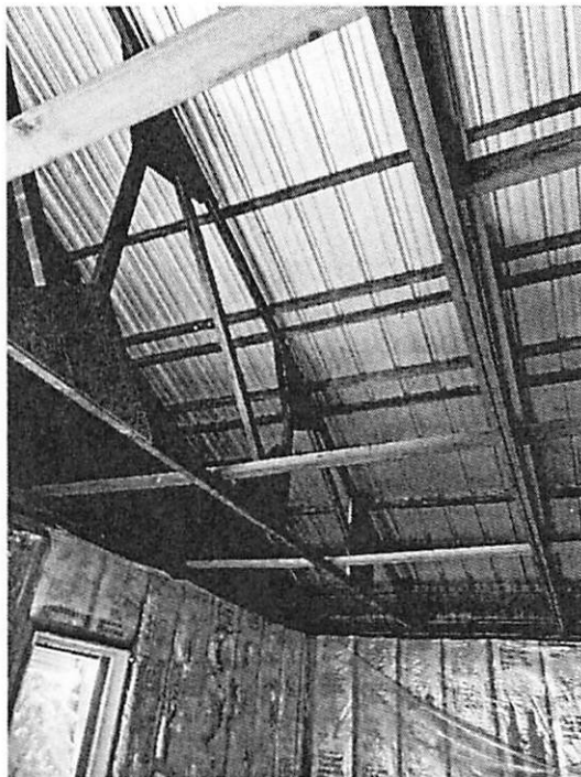
Photo 2: Site-Built Wood Truss
