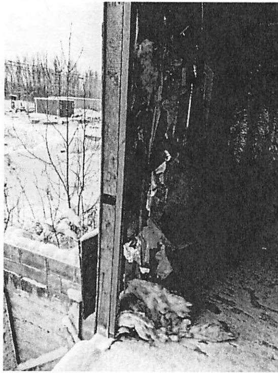
Photo 3: 2x4 wall with sistered 2x2
