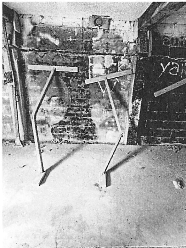
Photo 8: Buckling Wall Brace
