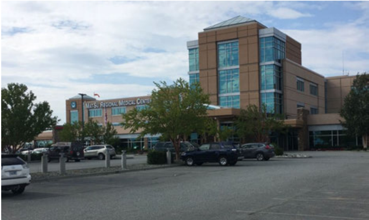
Figure 15. Mat-Su Regional Medical Center
