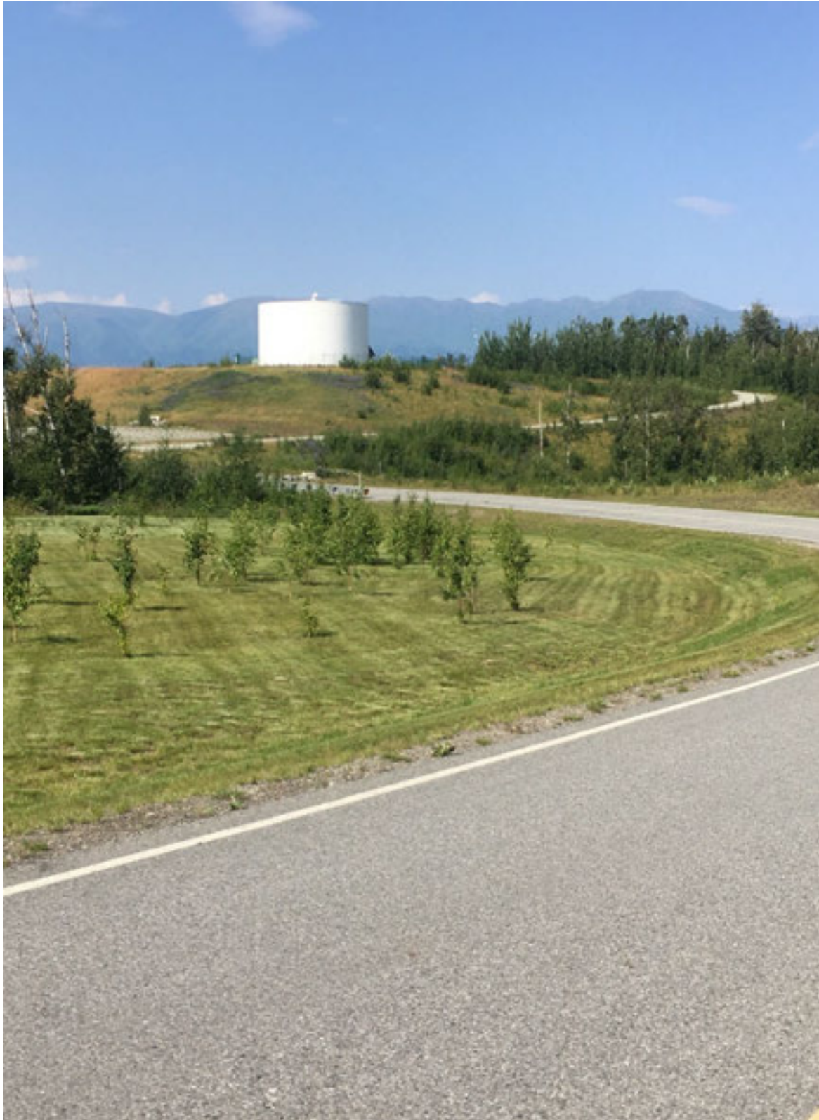
Figure 14. City of Palmer Water Reservoir Located at East College Drive and North Trunk Road
