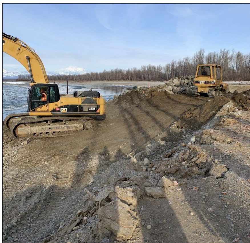
Figure 12. Emergency rock placement occurring along dike extension in 2020.
