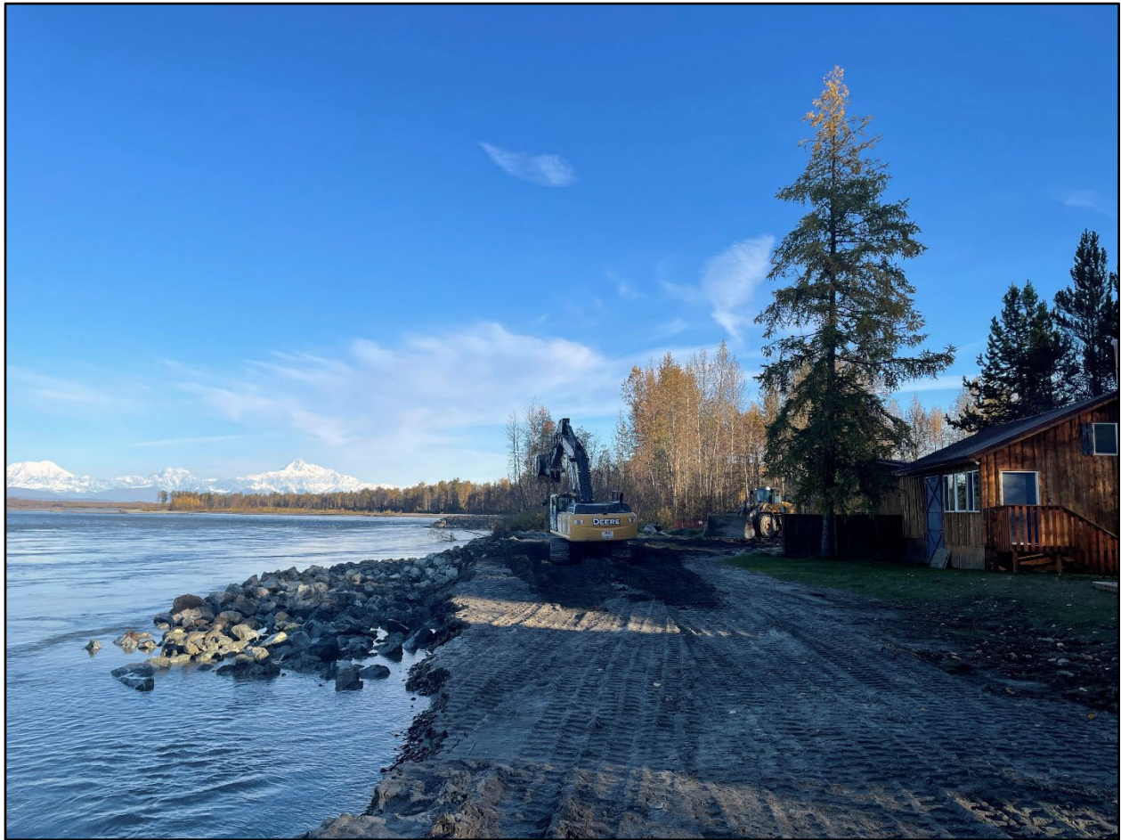
Figure 16. Emergency placement of revetment material following early September 2023 flood event.
