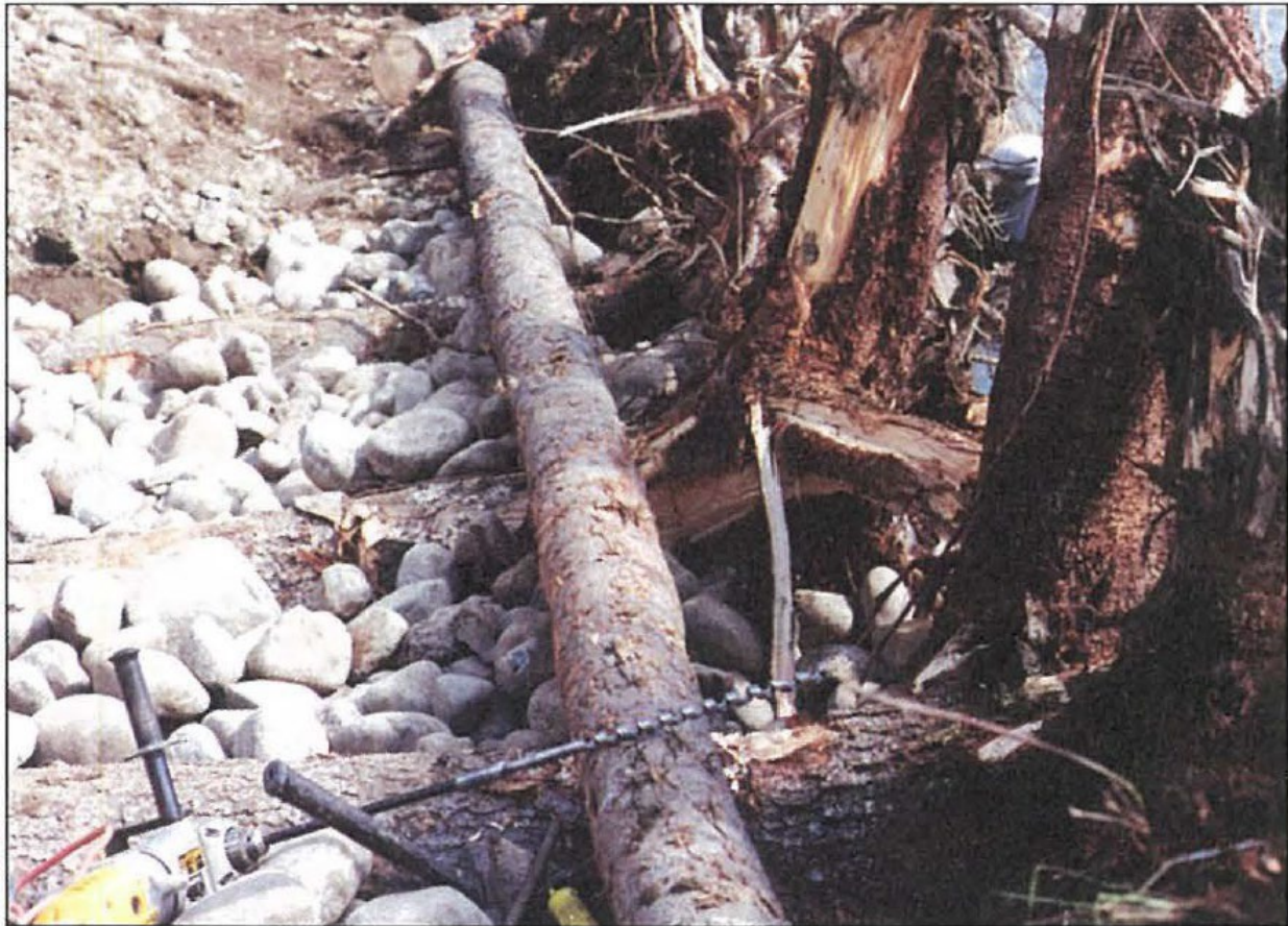
Figure 26. Root wad revetment construction (rock layer with header log pinning) at Pioneer Lodge in Willow Creek, Alaska (Walter & Hughes, 2005).
