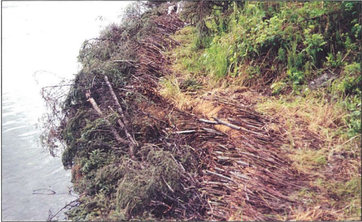
Figure 28. Cabled spruce trees and brush layering immediately after installation, Ciechanski Recreation Site, Kenai River, Alaska (Walter & Hughes, 2005).
