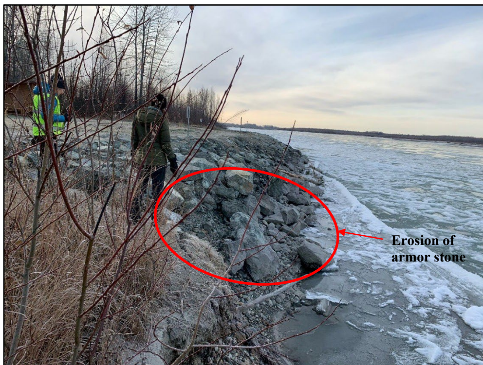
Figure 11. Erosion of armor stone along revetment observed in 2020.
