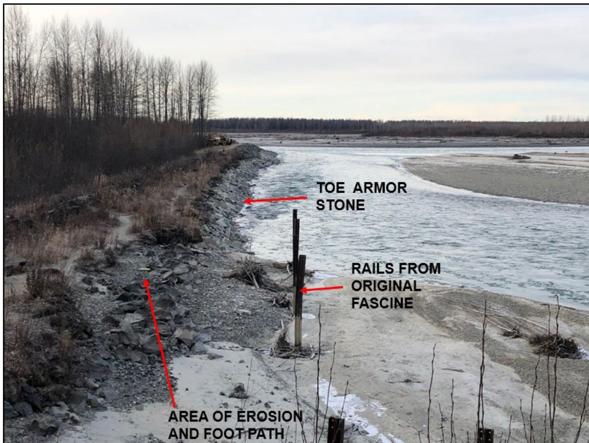
Figure 10. Erosion of dike observed during low water in 2020.
