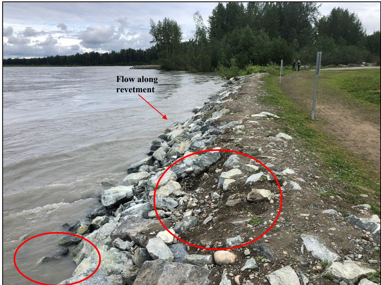
Figure 9. Erosion and loss of armor stone observed along revetment in 2021.
