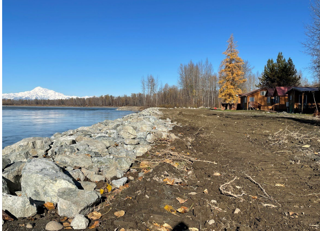
Completed revetment as seen from south end of repair on 10/4/23.
