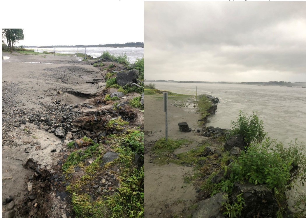
Photos of revetment damage taken on the evening of 9/5/23
