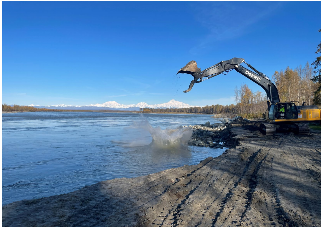
Riprap installation in revetment repair zone.
